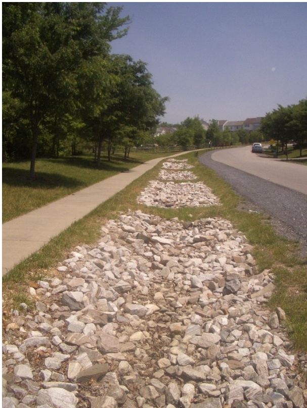
Rural Highway Infiltration Subsurface
