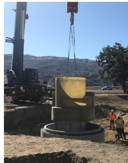
Example Hydrodynamic Separator
