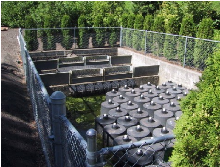
Example Cartridge Media Filter
