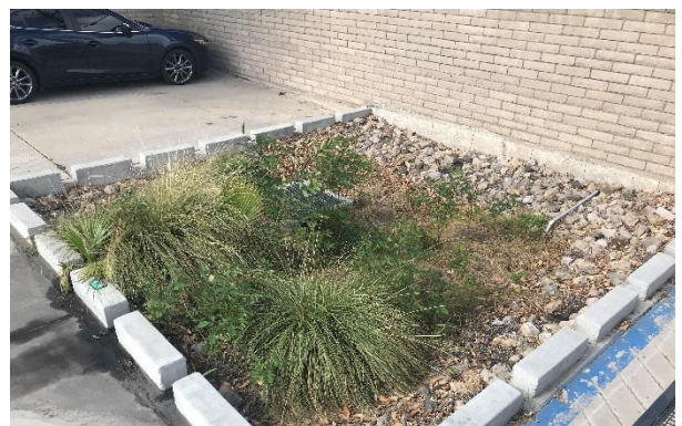
Biofiltration in Parking Lots
