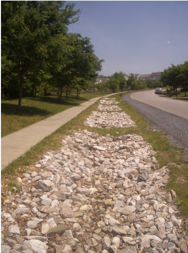
Rural Highway Infiltration Trench
