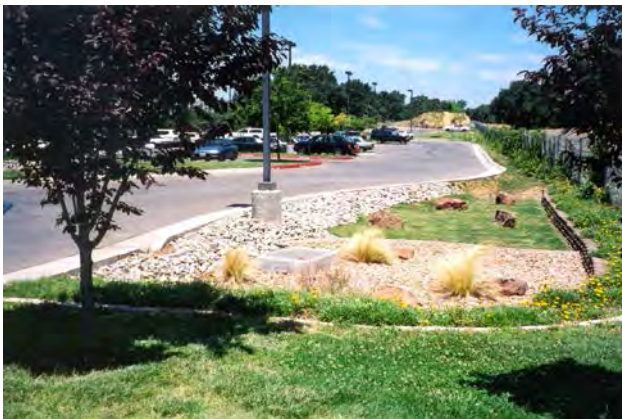
Sand filters connected to impervious surfaces
