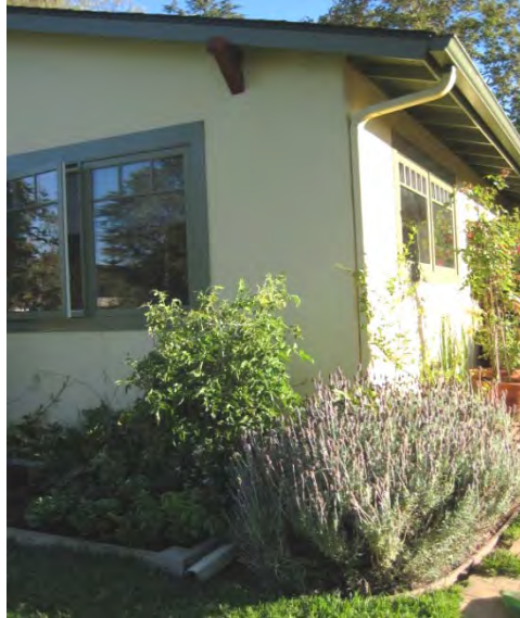
Diverted Roof Runoff City of Santa Barbara
