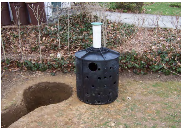
Drywell installation
