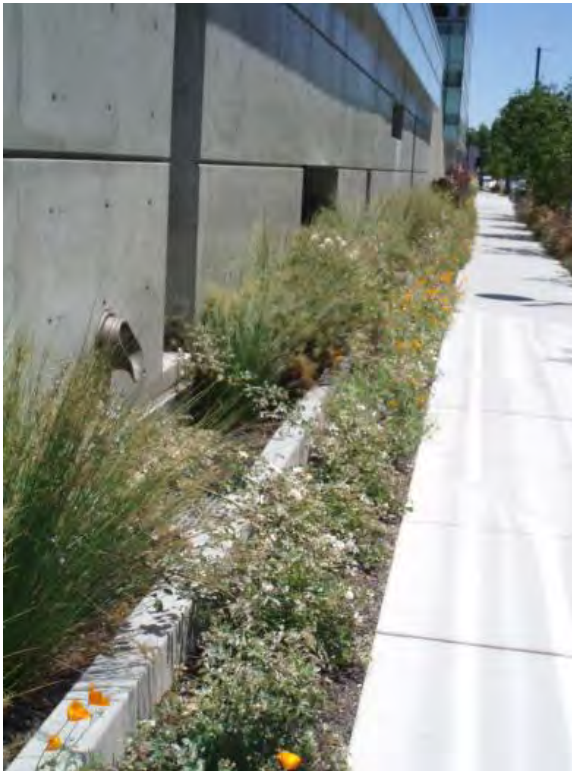
Planter boxes extending along a building wall
