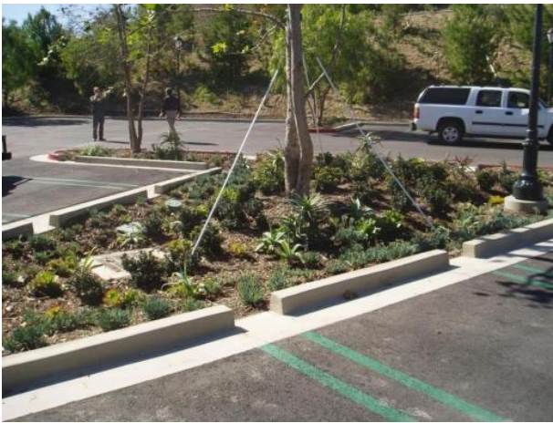
Bioretention in Parkway and parking lots
