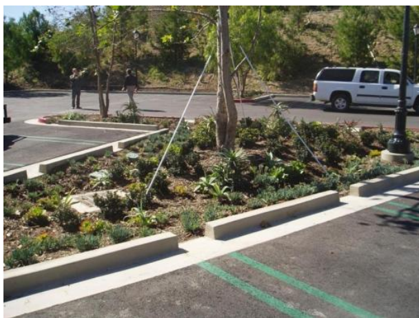
Bioretention in Parking Lots
