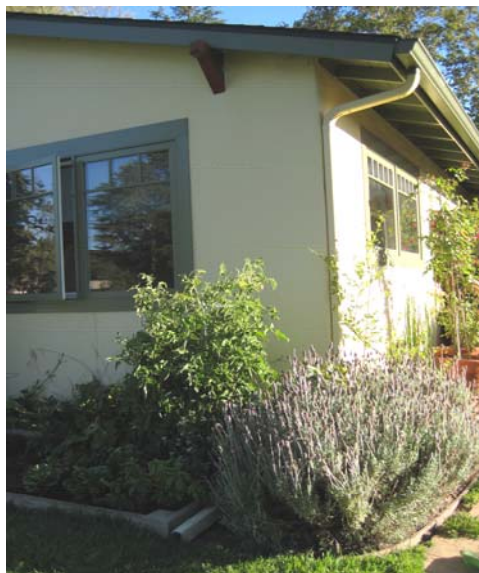
Diverted Roof Runoff City of Santa Barbara
