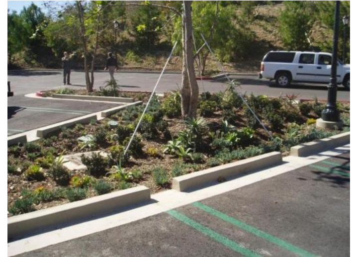
Bioretention in Parkway and parking lots
