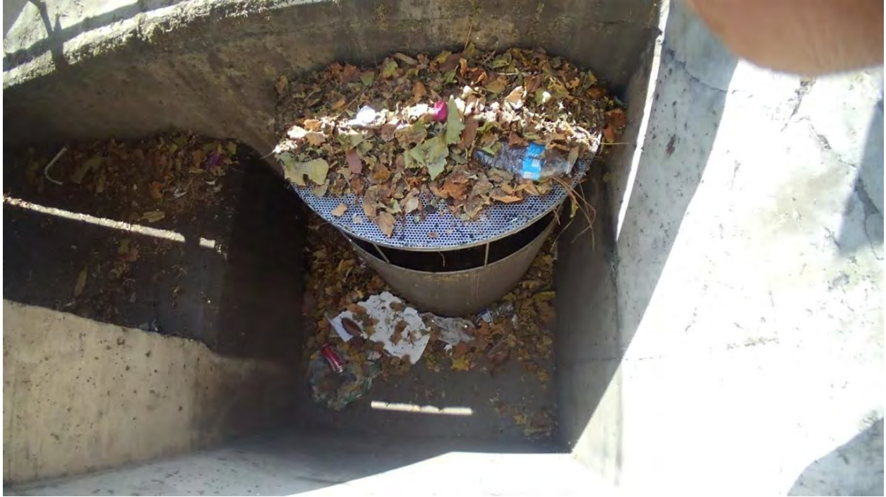
Figure 1: Catch basin prior to cleaning (City of Camarillo catch basin)
