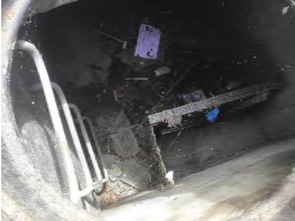
Figure 3: Catch basin prior to cleaning (County of Ventura catch basin)
