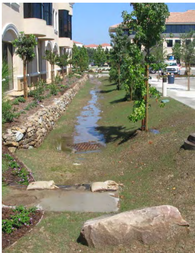
Low Impact Development BMP
