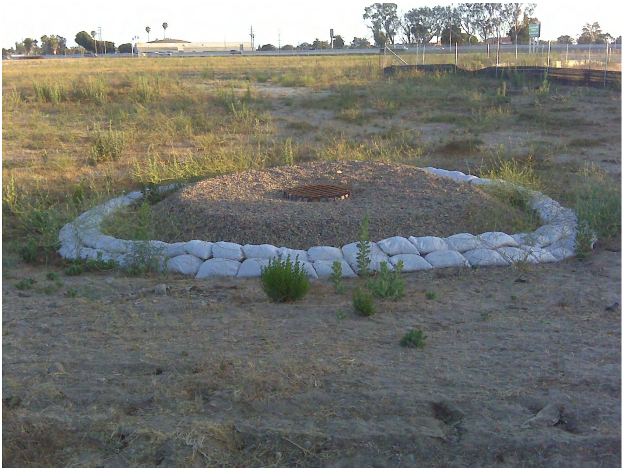
Storm drain protection during construction
