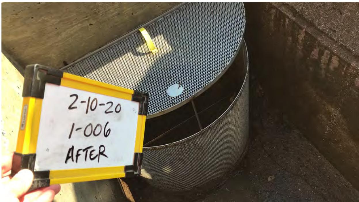
Figure 2: Cleaned catch basin (County of Ventura catch basin)
