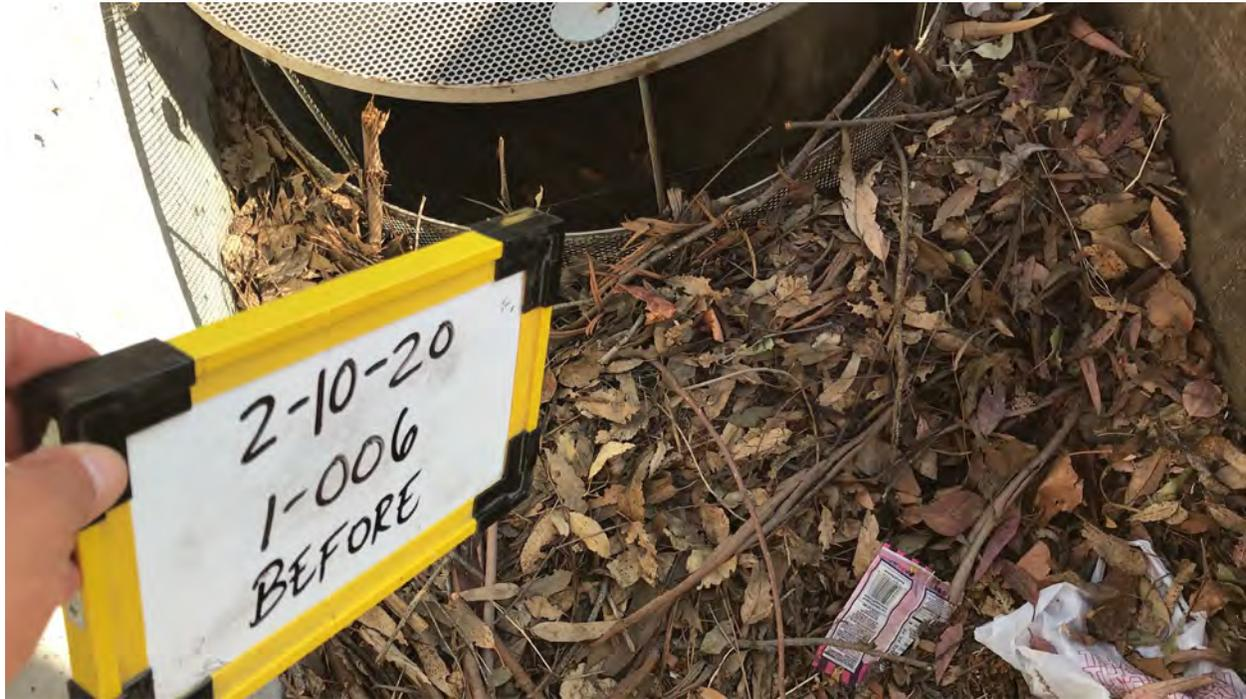
Figure 1: Catch basin prior to cleaning (County of Ventura catch basin)
