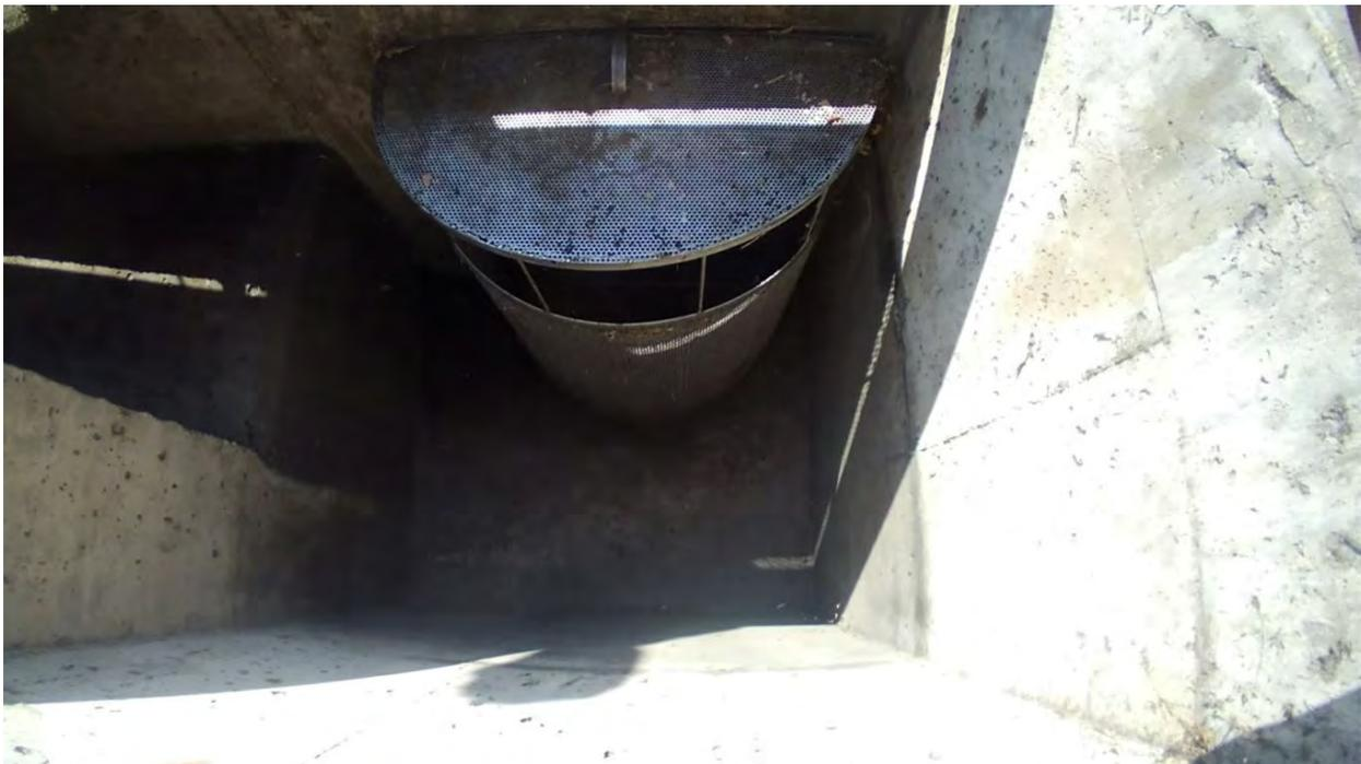
**Figure 2: Cleaned catch basin (City of Camarillo catch basin)**
