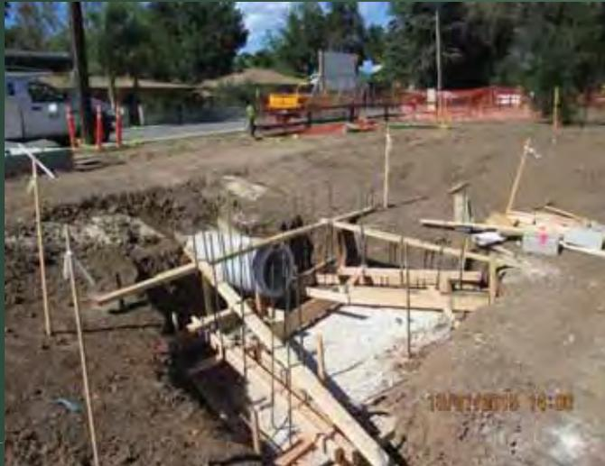
Constructing concrete headwall
