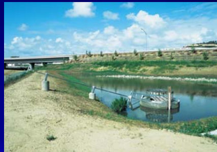
Extended Detention Basin
