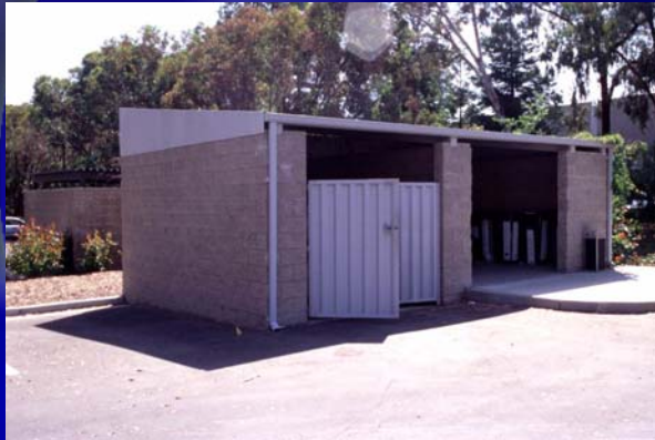
Outdoor Trash/Material Storage Area
