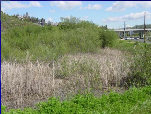
Poorly Maintained BMP
