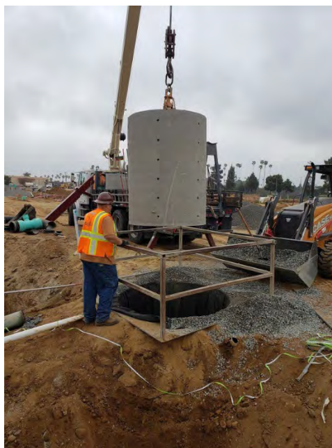
Drywell Installation
