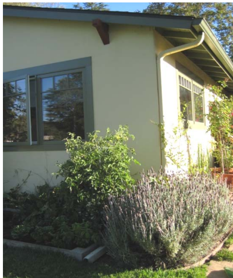
Diverted Roof Runoff City of Santa Barbara
